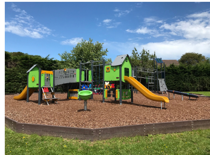
Play area renewal at Lower Brook Drive, Ivybridge
